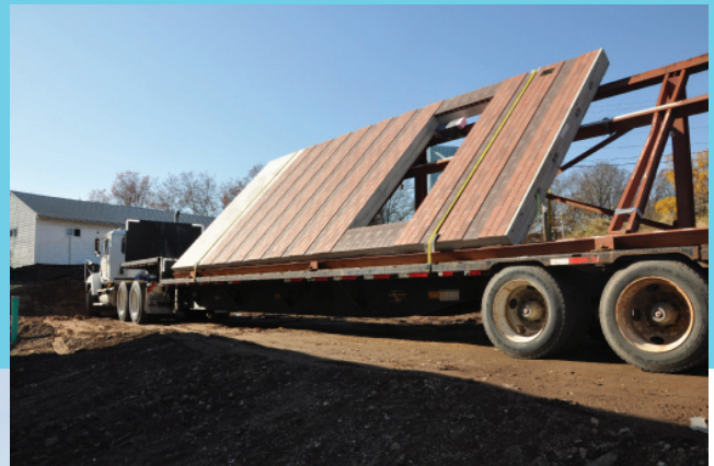
Pre-cast exterior concrete panels are manufactured off site and trucked into the building site then dropped in place using a heavy-duty crane. Photo Credit: Dan Desmet, Public Affairs
